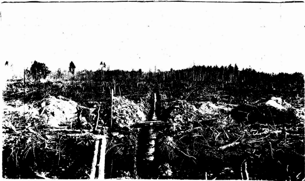
One of the Lateral Ditches
