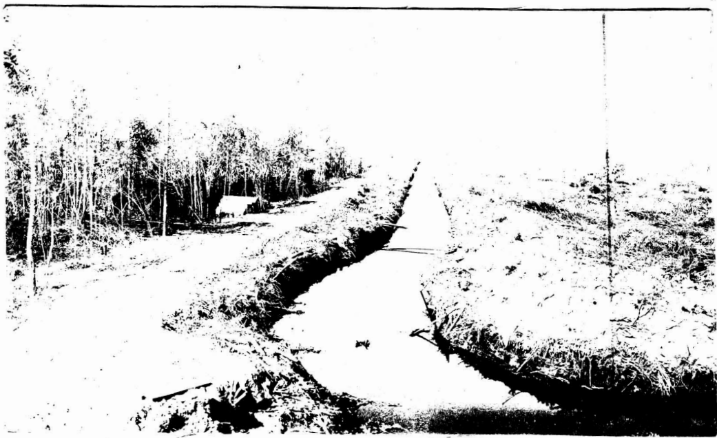
One of the Main Drainage Canals
