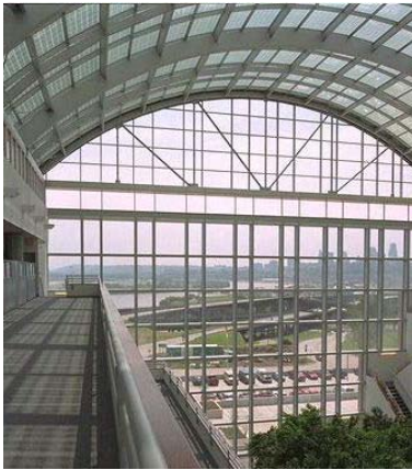
Figure 3. Atrium at the U.S. EPA Regional Headquarters, KS The atrium design provides most of the office space with natural light. The atrium's glass has a low emissive coating, receiving daylight while reflecting large percentages of the infrared spectrum, which controls heat gain (Whole Building Design Guide, 2005).
