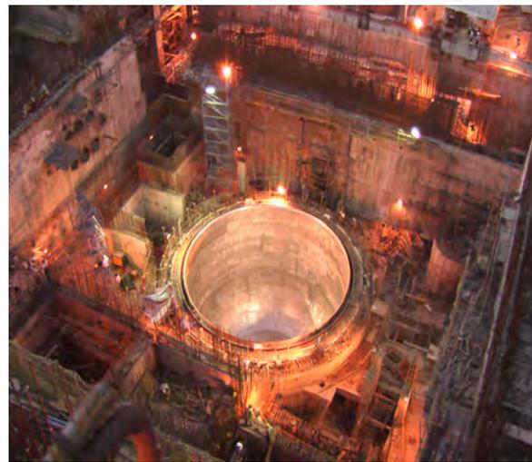
Fig.5 Successful erection of safety vessel on the inner wall of reactor vault
