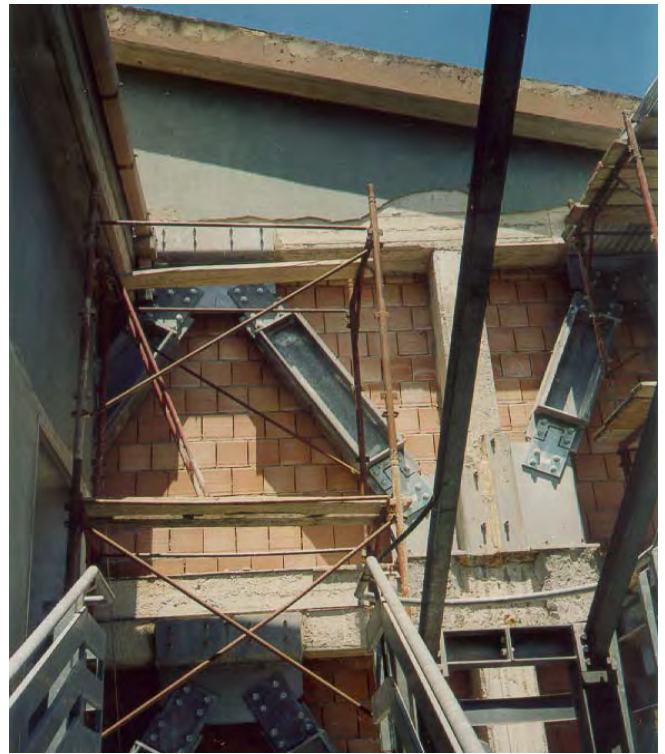
Figure 3: Visco-elastic dampers installed in the Gentile Fermi school at Fabriano (a rare example of rationalist architecture), during seismic improvement works (filmed in 2001).
