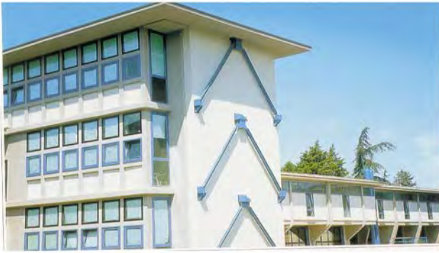
Figure 3: Visco-elastic dampers installed in the Gentile Fermi school at Fabriano (a rare example of rationalist architecture), during seismic improvement works (filmed in 2001).
