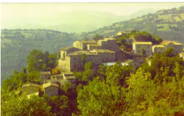
Figure 7a: View of the village of Mevale di Visso (Macerata) after the restoration performed to repair the serious damage caused by the Valnerina earthquake in 1979.
