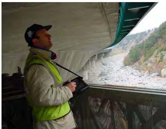
Fig.5: Site inspection using pen-touch computers
