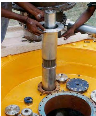
Fig. 9 Removal of tested IHX
