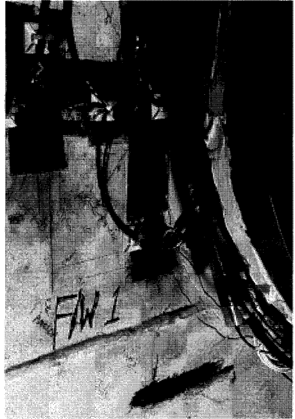
Figure 9 Liner Tear at Locations 15 (Equipment Hatch) and 3 (Feedwater Penetration)
