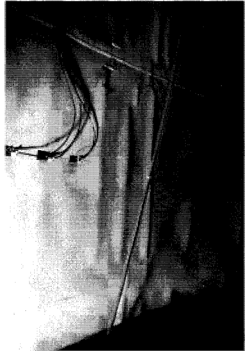
Figure 11 Liner Buckling
