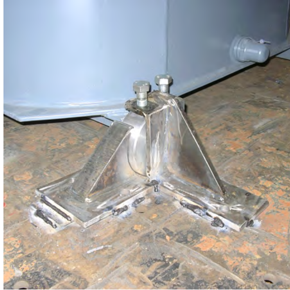
Fig. 9 Additional fixing devices for wheels
