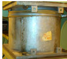
Fig. 2 Spring-damper system for the EDG set
