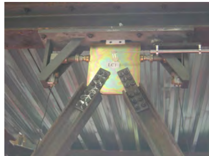
Fig. 3 - View of a Jarret viscous fluid damper
