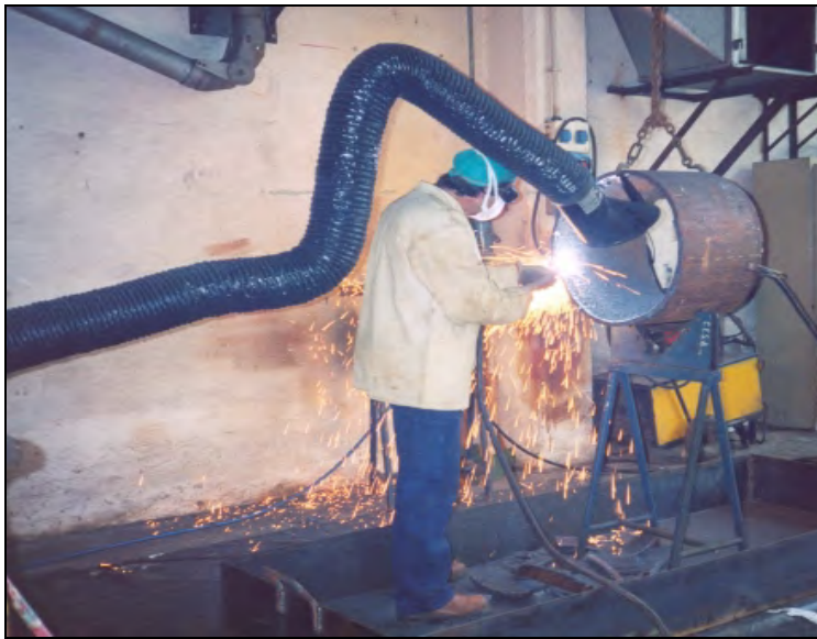
Fig. 5 Plasma torch cut of a 30" piping spool
