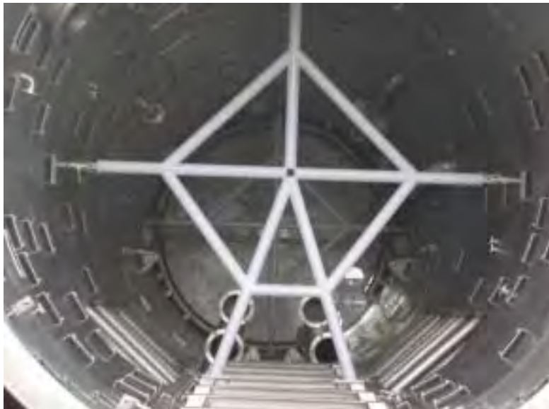
Figure 13: Reinforcements structures for the hydrostatic test
