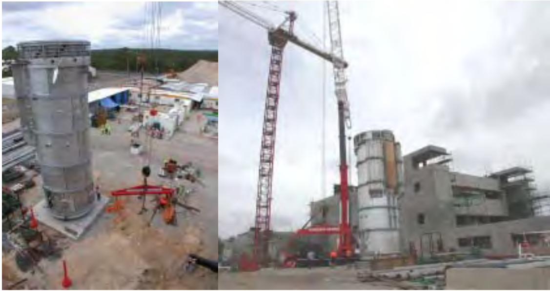
Figure 4: Reactor Pool completed next to the reactor building
