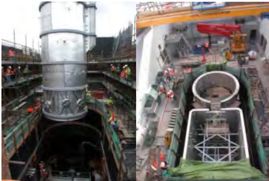
Figure 20 – Lifting and installing the reactor and service pool
