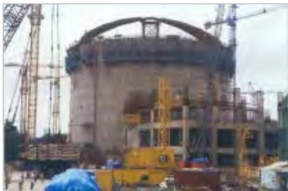
*Fig.7 Erection of dome formwork supporting structure*
