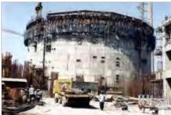
*Fig.5 - IC wall - Automated self- climbing formwork system*
