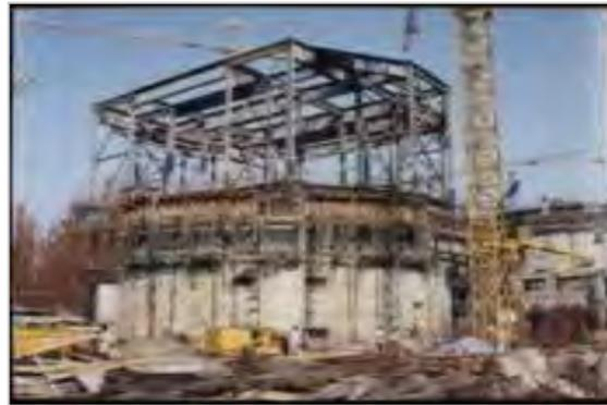
*Fig.4 -Reactor building internals- structural steel framework*
