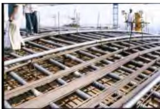
*Fig.9- Layout of prestressing cables in dome*
