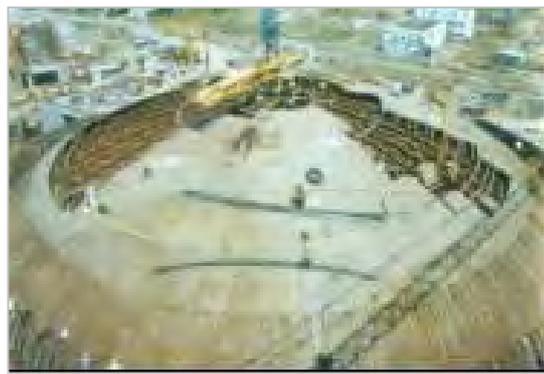
*Fig.8 Dome formwork fixing*
