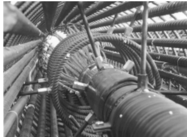
Fig. 8 The reinforcement and the prestressing of the experimental piles ([11])
