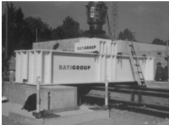
Fig. 7 Testing site for determination of the tensile capacity of bored piles ([11])
