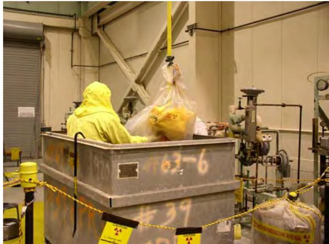
*Fig. 3. CRDM muzzle assembly being removed from shipping container.*
