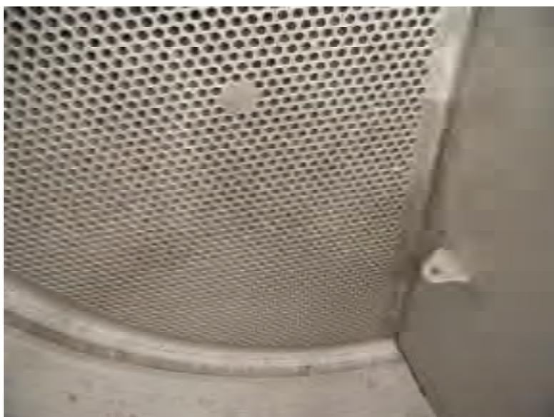
Figure 4: SG Channel Head with Tube Sheet after Decontamination
