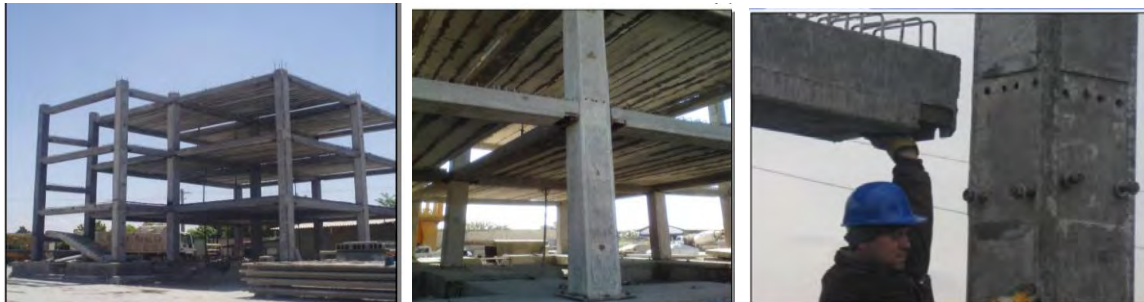
Figure 1, Structural assembling process
