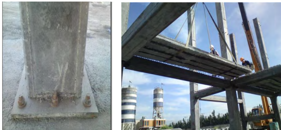
Figure 3, Base connection and flooring system
