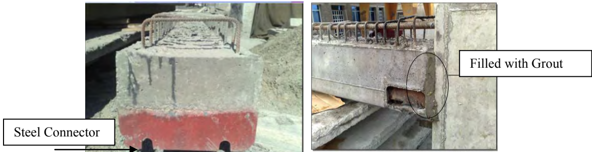
Figure 2, Structural assembling process
