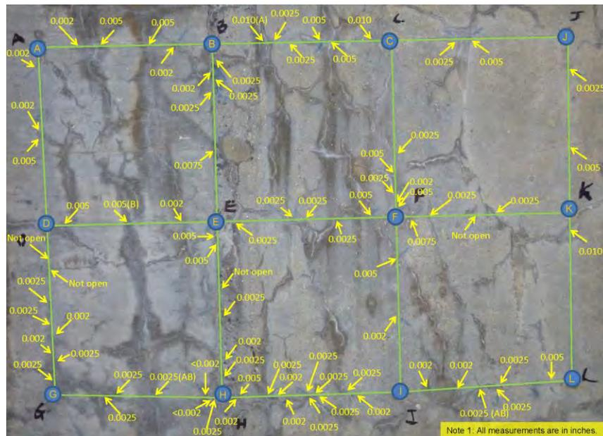
Figure 7. Crack widths and the crack location at an ASR Monitoring Location
