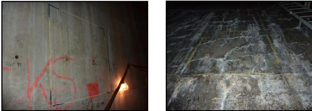
Figure 4. Examples of visual rating of ASR distress on CEB Wall (Left: 1; Right: 4)
