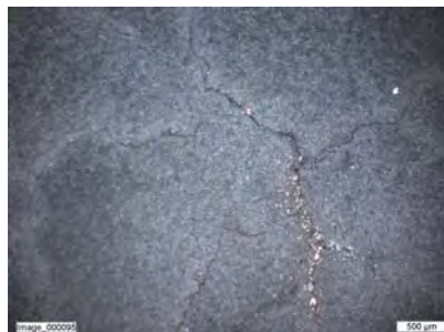
Fig. 11e: Crack network after 525 \cdot 10^3 cycles top side surface.
