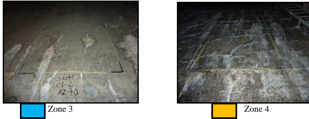
Figure 4. Photographs of ASR Visual Rating Zones
