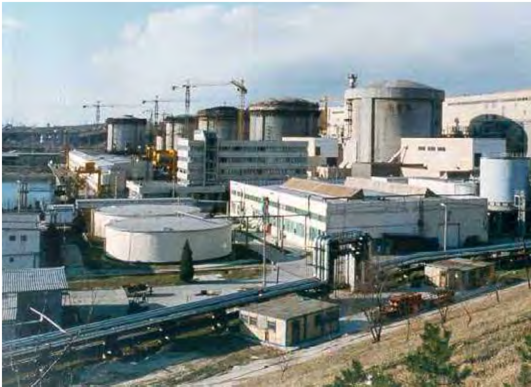
Figure 1. View of Cernavoda Nuclear Power Plants
