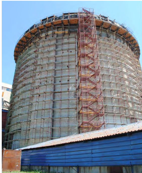
Figure 2: Scaffolding Arrangement Around Containment Wall
