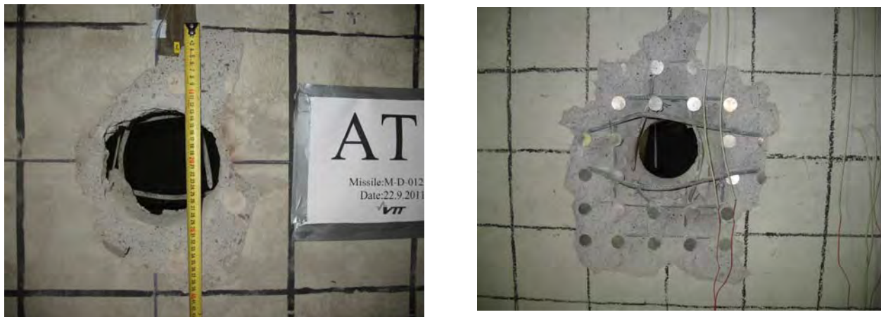
Figure 5 Front and rear side of the slab with longitudinal reinforcement and transverse reinforcement in form of T-headed bars after the test
