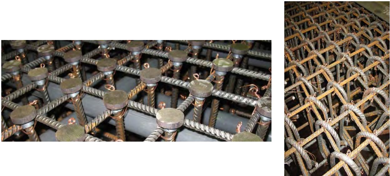
Figure 2 Transverse reinforcement in form of T-headed bars (above) and conventional stirrups with 180 degree hooks (on the right)
