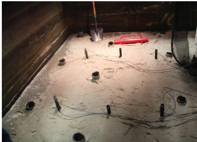
Figure 3a. Pile foundation installed
