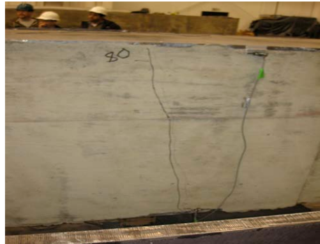
Figure 9. Cracking of OOPV+T-3.5 under combined axial tension and shear loading
