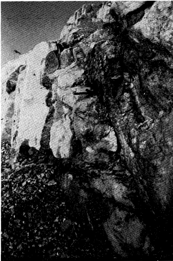
Figure 4C North wall of Falls Reservoir spillway showing traces of three major joints.
