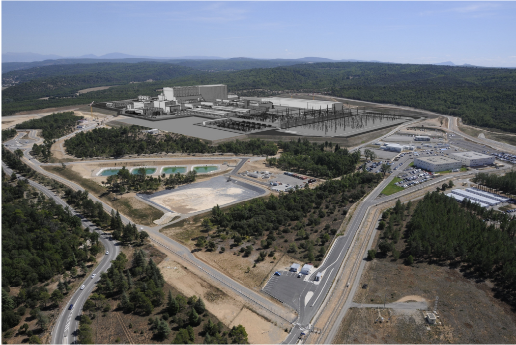
Fig. 1: Birds Eye View of ITER Facility
