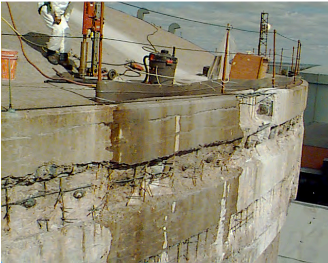
a) Before repair, 1999
