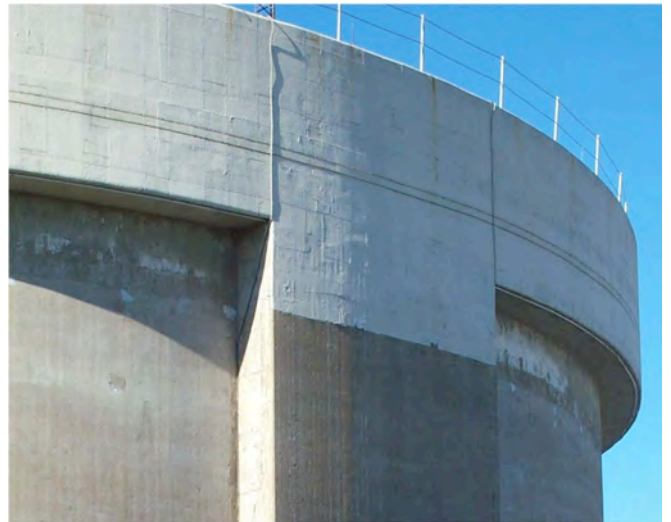
b) After repair, 2008
