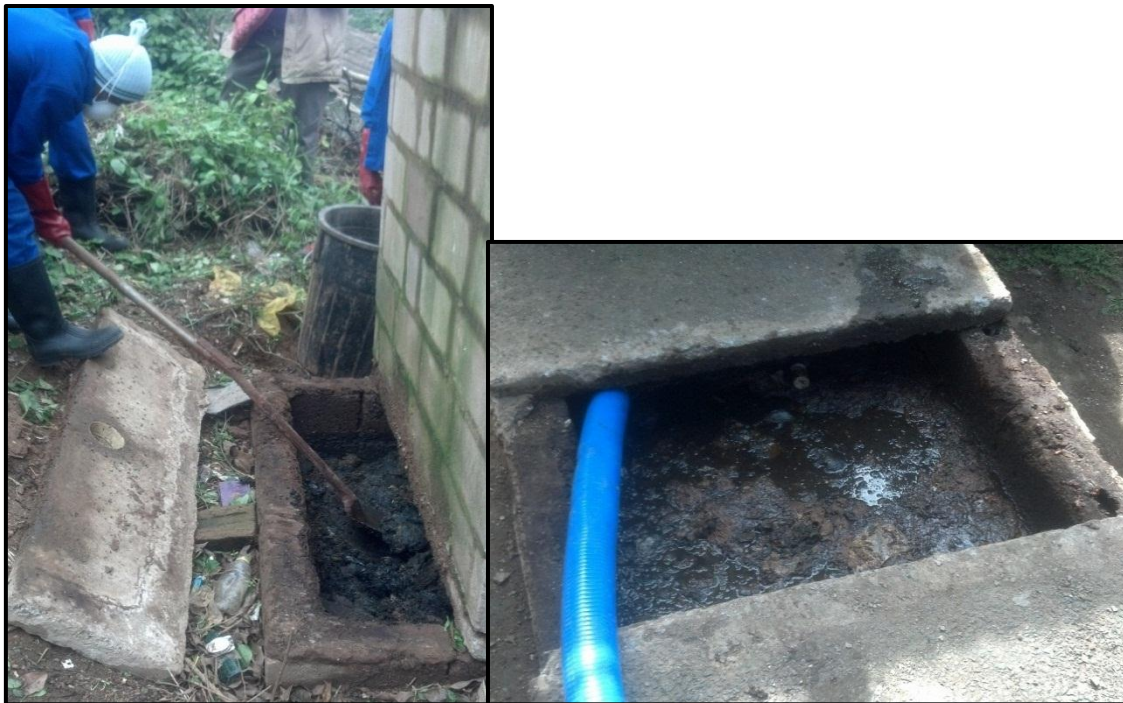
Figure A.6 A “dry” pit latrine (left) and a “wet” latrine (right) found less than one mile apart.
