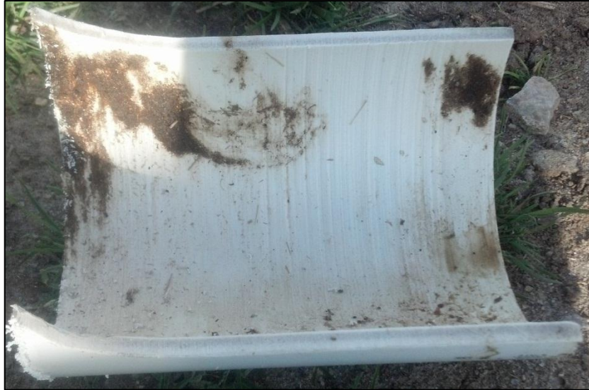
Figure C.7 Deterioration of a section of pipe after testing with the hydraulic motor in dairy waste.
