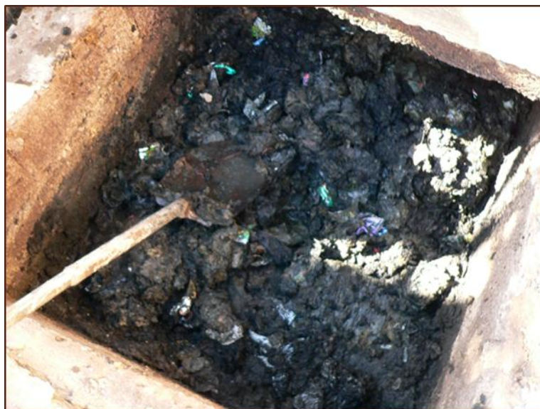
Figure A.7 Pit latrine with high solid waste content near Durban, South Africa (Photo: Buckley et al.).
