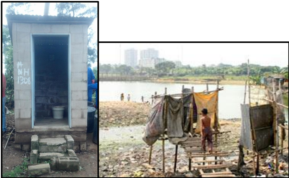
Figure A.2 An example of an improved sanitation facility, the Ventilated Improved Pit latrine (left). An example of an unimproved sanitation facility, a hanging latrine (right) (Photo: Wateraid / Abir Abdullah).
