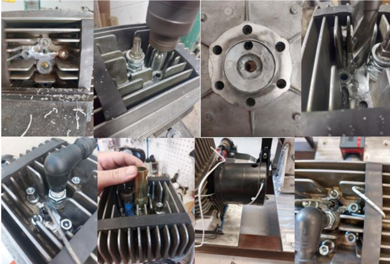
Figure 3.26: In-Cylinder Pressure Sensor Installation
