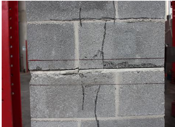
Figure 4.2 - Crushed CMU at Compression Face of Control Wallette at Failure
