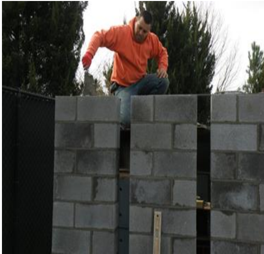
(c) Grouting Concrete
