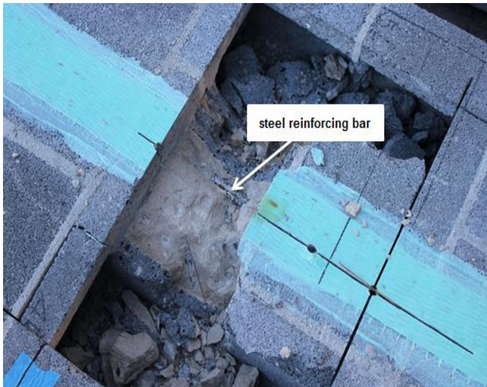
Figure 4.53 - Location of Steel Reinforcing Bar in GS3-1
