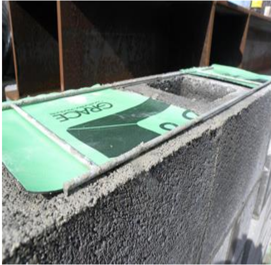
(a) Joint Reinforcement
