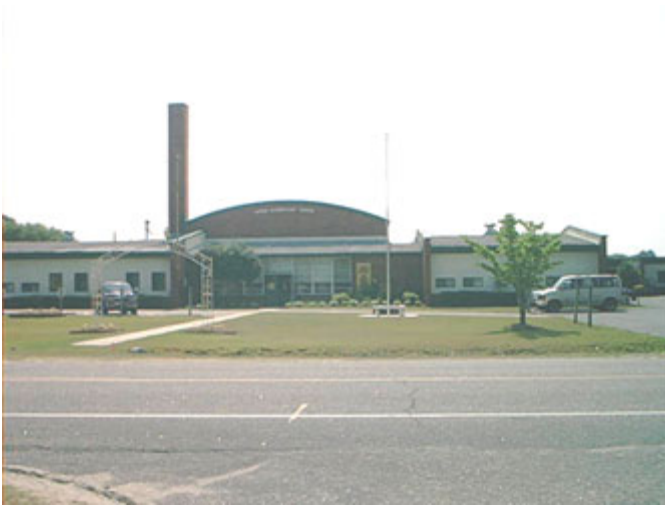
Figure 11. Union Elementary School 9
