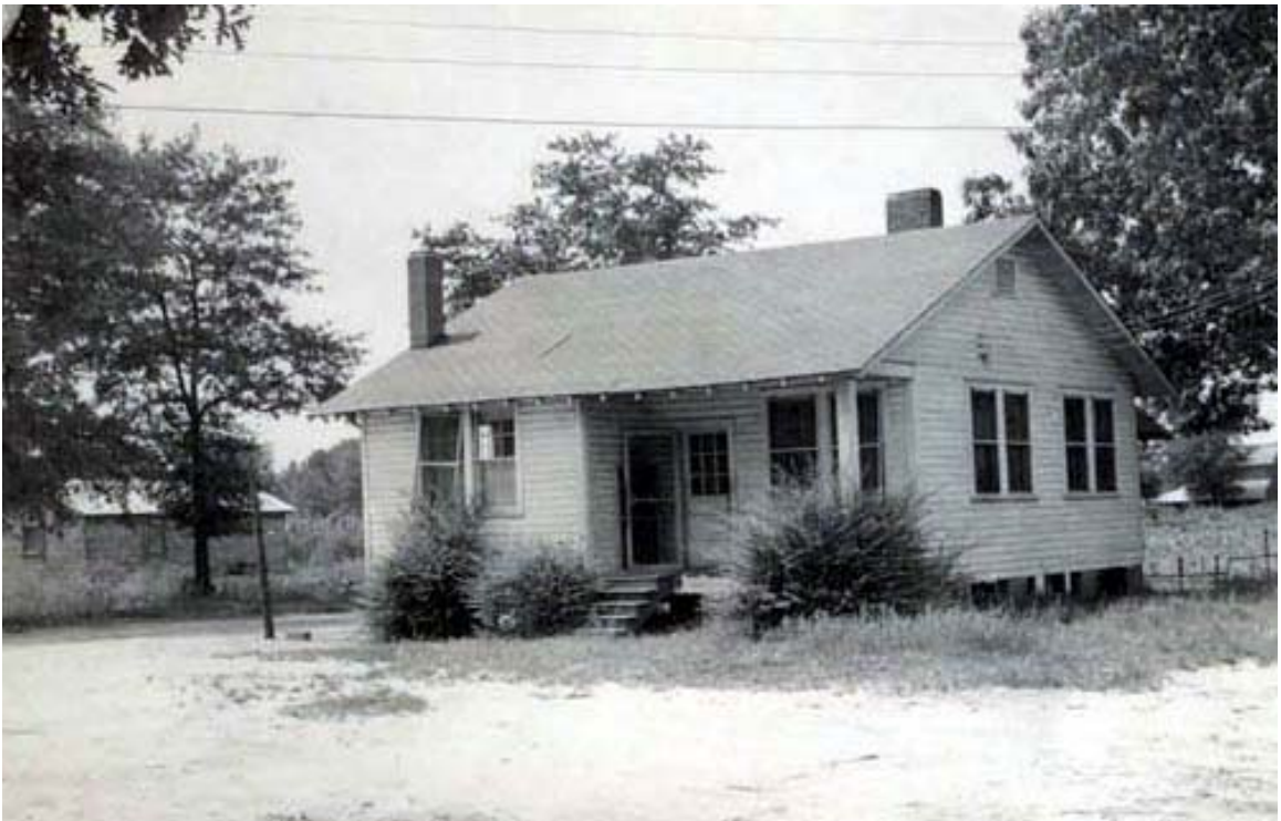
Figure 9. Green Grove High School Home Economics Building 7
