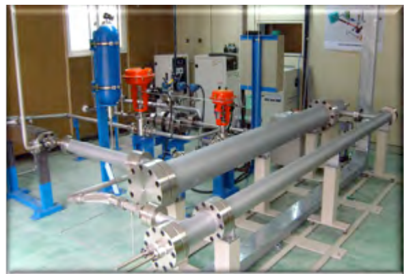
Fig.3 Photo of primary nitrogen loop
