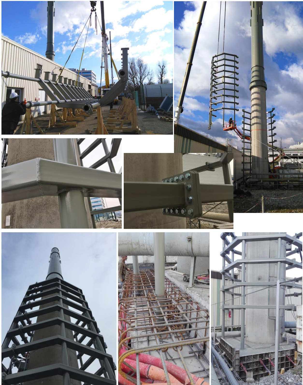
Figure 9. Construction of stack shield.
