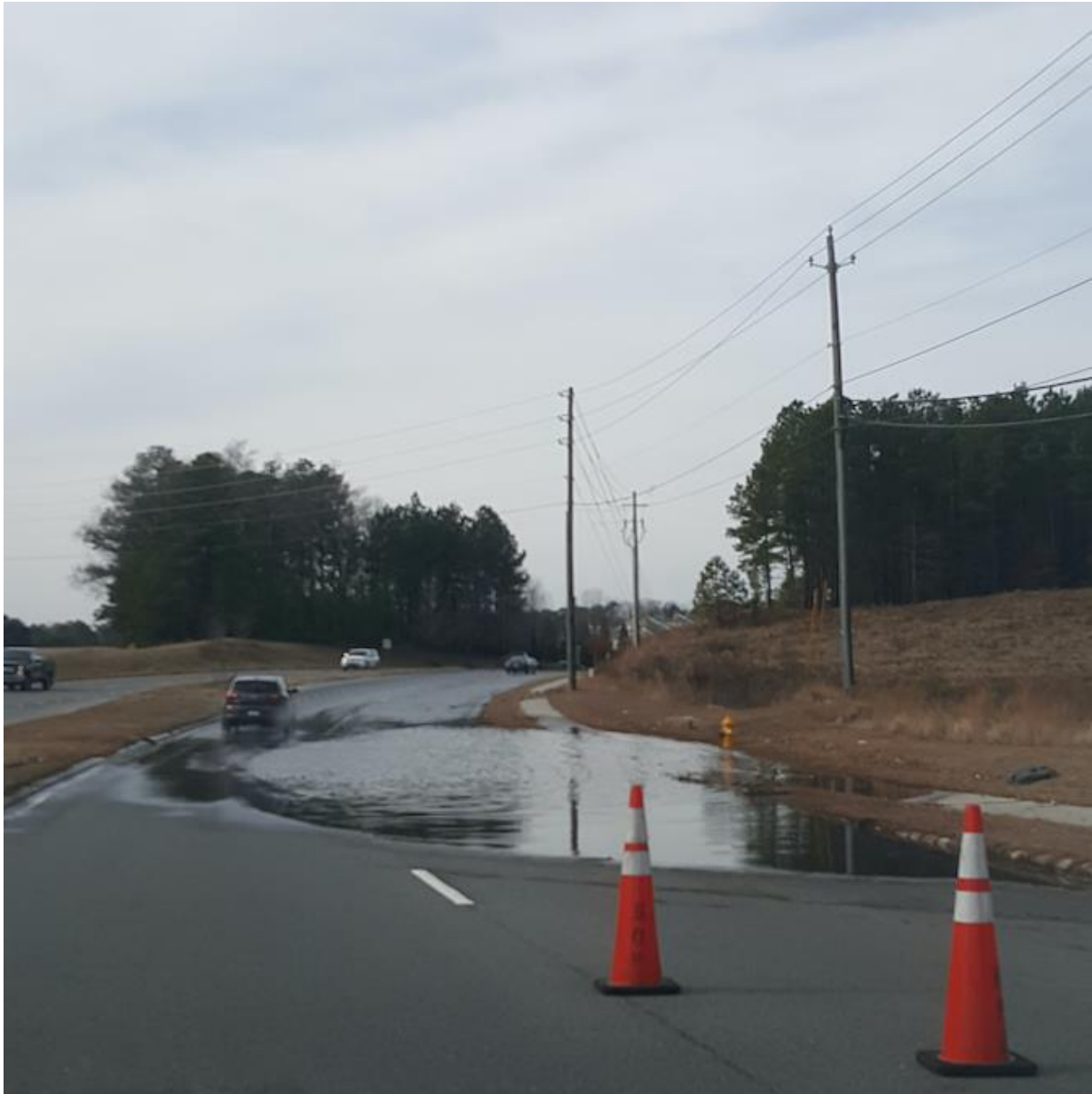
Figure 2.1 Flooding in the watershed. Cars drive through a flooded portion of the road in the Walnut Creek watershed days after a hard rain.
