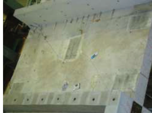
Figure 8: Ultimate state of the floor - Model-1 (after unloading; cracks partially closed)
