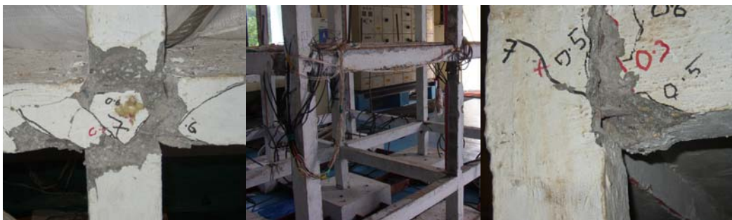
Fig 12 Damage patterns in Joints
