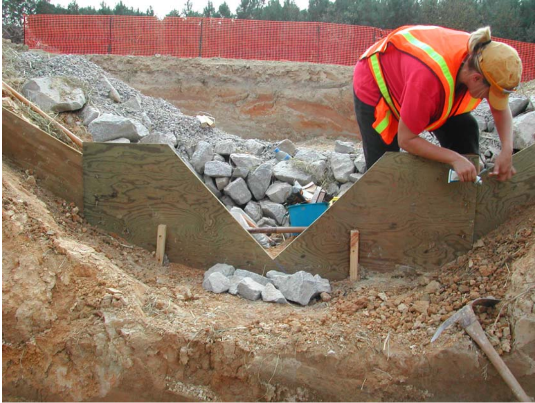
Figure 9. End contractions installed on both ends of the weir to ensure flow diversion and to reduce erosion on side walls.
