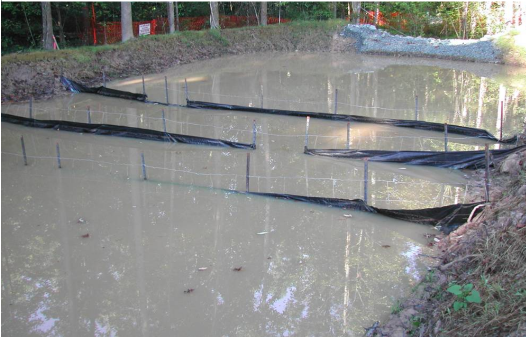
Figure 2. Silt fence used as baffles. Weirs were cut on opposite sides to increase the flow path as runoff moves out.
