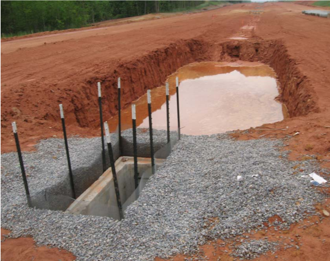
Figure 11. Standard 10-year Trap with standing pool with spillway entering culvert pipe that runs under road bed
