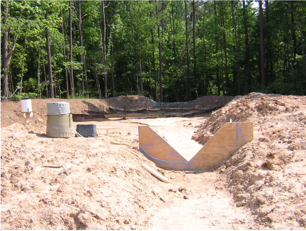
Figure 17. Standard Basin with Silt Fence Baffles at the onset of monitoring.
