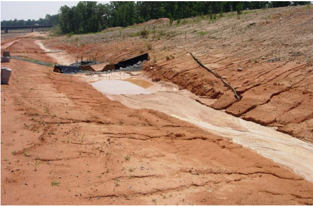
Figure 8. Upslope image of Standard 10-year Trap14 showing the ditch line modification and samplers installed on the left hand side.
