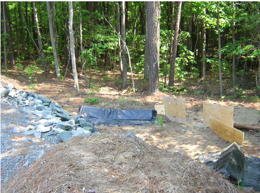
Figure 18. Standard Basin with Silt Fence Baffles exit was installed with a rectangular weir to monitor flow.
