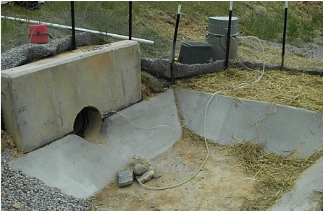
Figure 14. 15 inch culvert pipe exiting the basin and entering into a level spreader.
