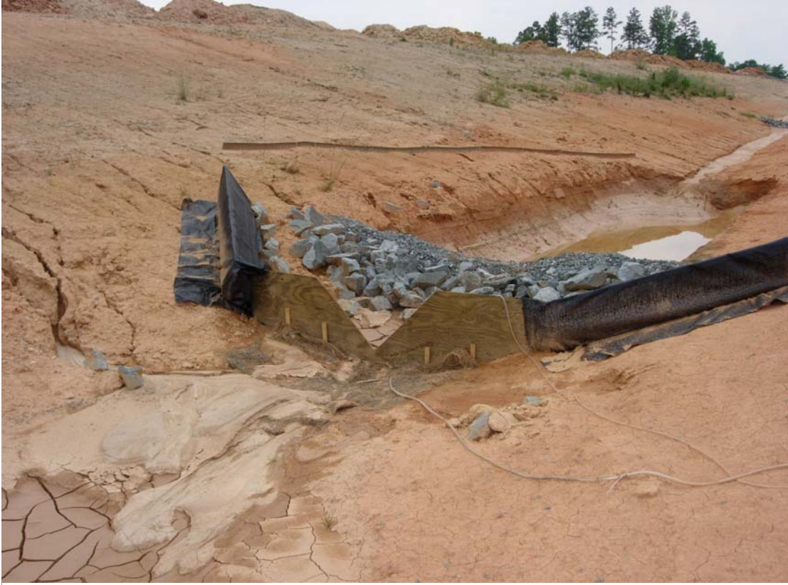
Figure 7. Standard 10-year Trap14 with a 90° V-notch weir installed on the downslope of the exit weir.
