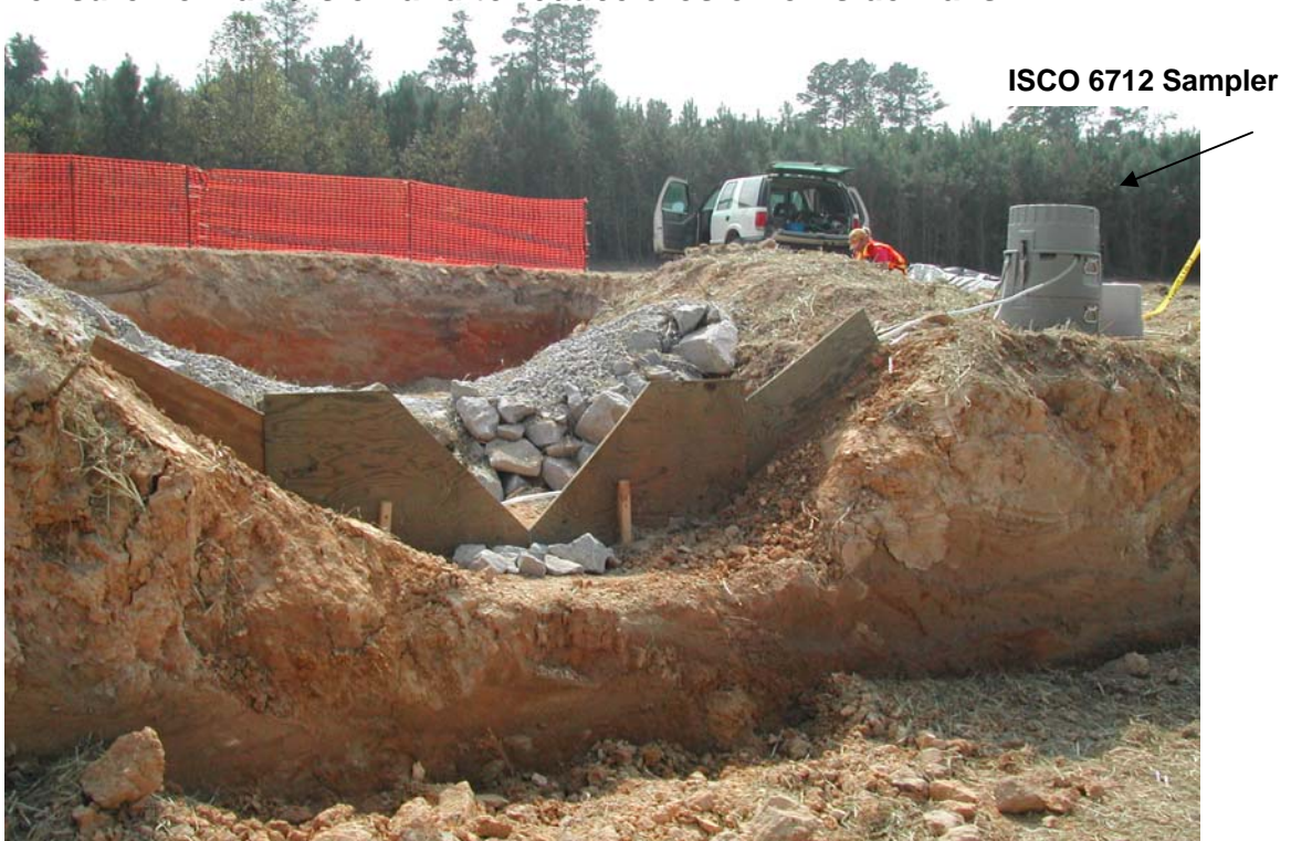
Figure 10. Standard 10-year Trap1 with a 90° V-notch weir installed behind the rock weir.
