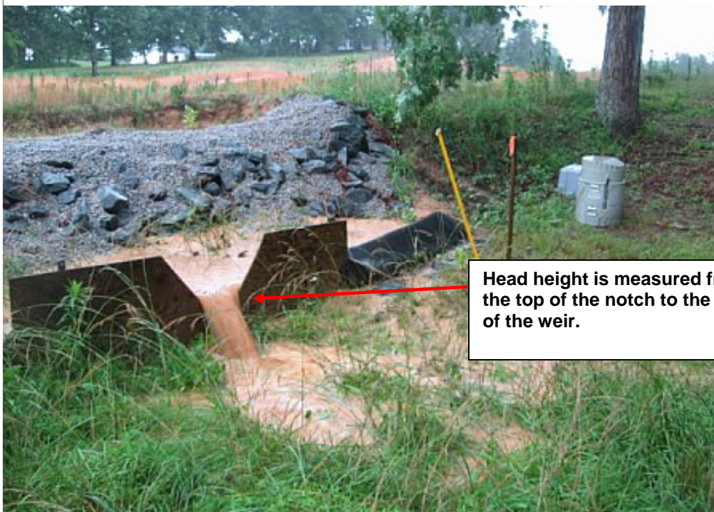
Figure 16. Standard 25-year Trap installed with a 90° V-notch weir with head height of 20 inches.
