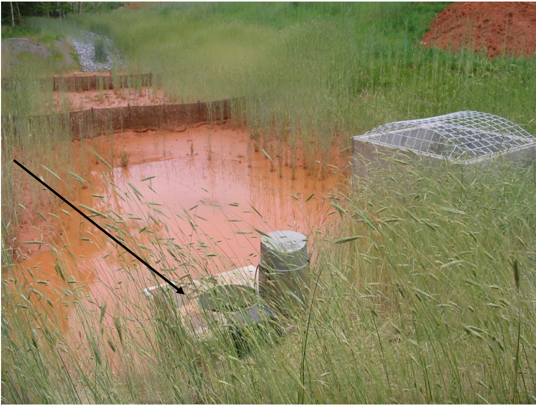
Figure 13. Skimmer Basin installed with a skimmer and emergency spill way.
