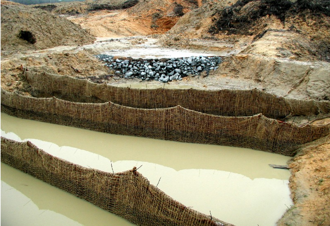
Figure 1. Porous baffles in a sediment basin. The flow is divided evenly across the basin to reduce turbulence and flow rates.
