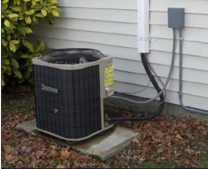
Figure 2. Conventional Heat Pump Outside Air Unit
