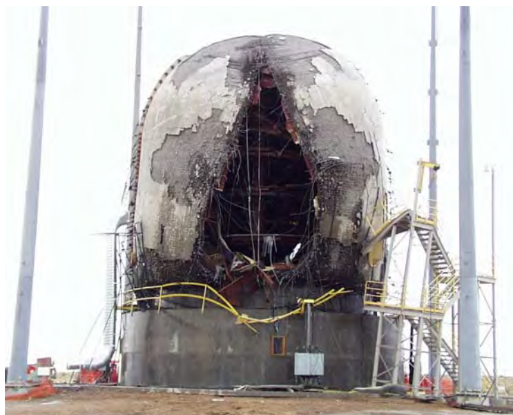
Figure 4 PCCV Model after the Structural Failure Mode Test
