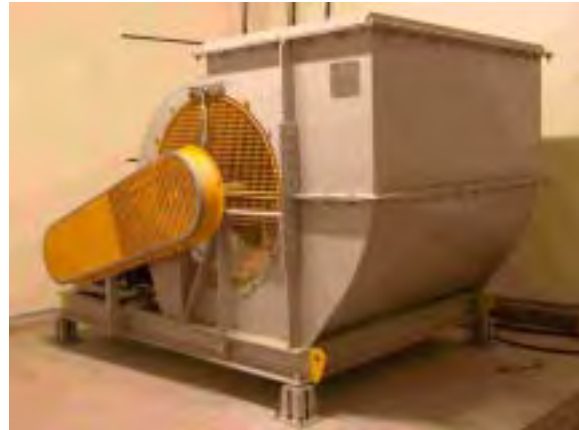
Figure 13 - Water Chiller with seismic isolators and reinforcements Fans with isolators
