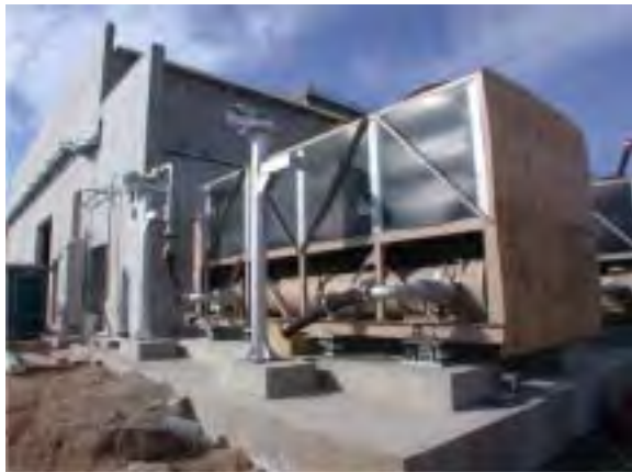
Figure 13 - Water Chiller with seismic isolators and reinforcements Fans with isolators
