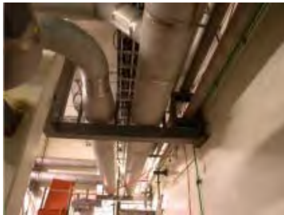
Figure 18 – Pipig Support
