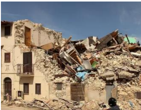
(a) L'Aquila building collapse
