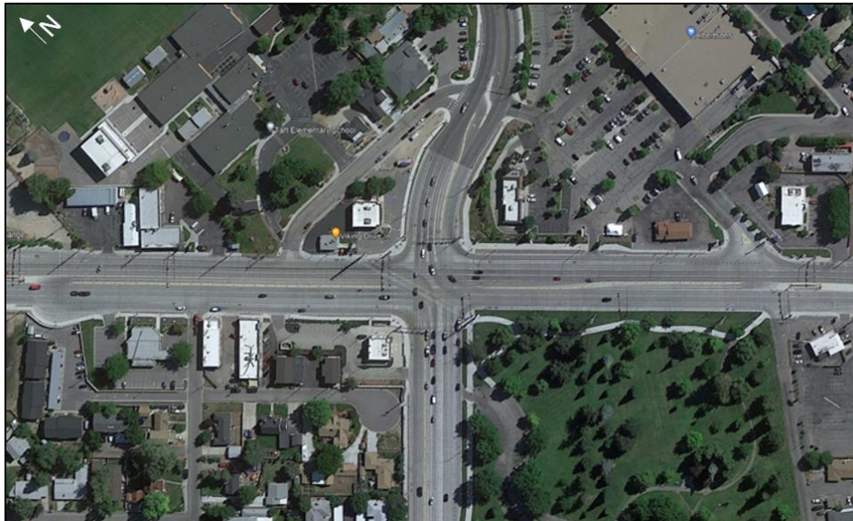
Figure 3. Partial MUT at State Street/Veterans Memorial Parkway, Boise, Idaho
