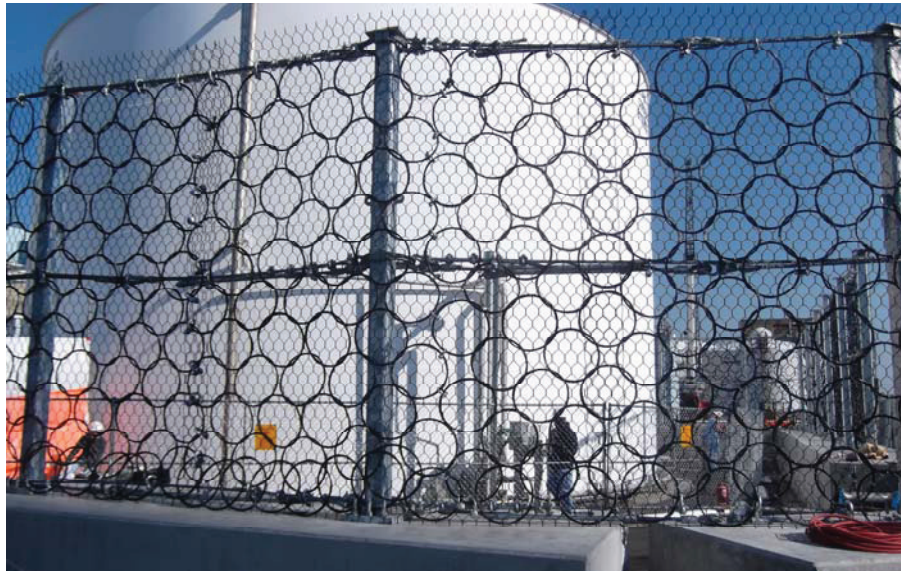
Figure 7. Photograph of Installed Perforated Barrier
