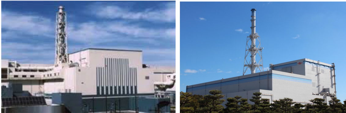
Figure 1: Stack Structures at Kashiwazaki-Kariwa & Tokai Daini NPPs (photos extracted from www.alamy.com )
