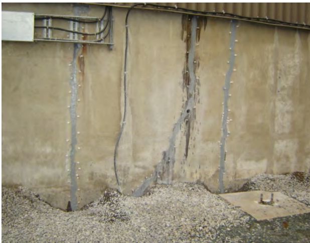
Figure 7 Epoxy Injection of Cracks in T/B Walls
