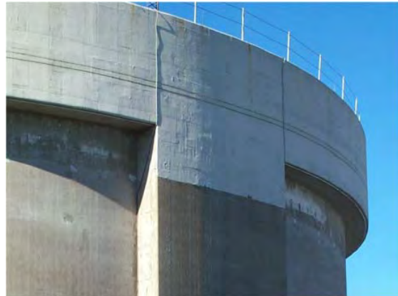
Figure 6 Condition of the Ring Beam After Repair
