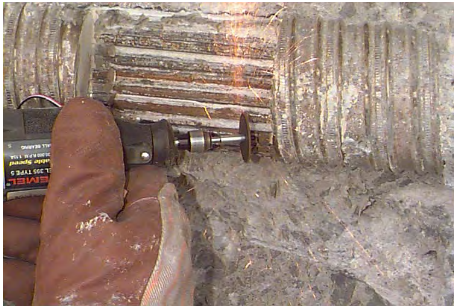
Figure 4 Inspection of Prestressing Cables
