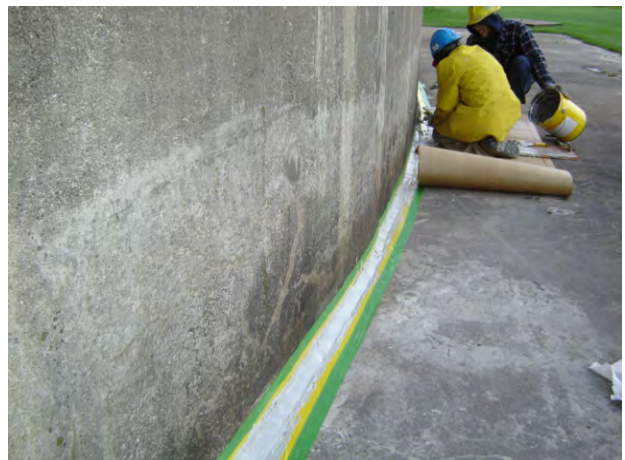
Figure 10 R/B Bottom Joint Sealant Repair
