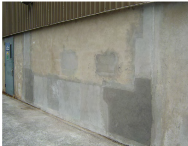
Figure 8 Repaired T/B Walls
