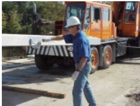
(a) Application of primer and epoxy
