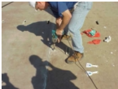
(c) FRP dowels installed
