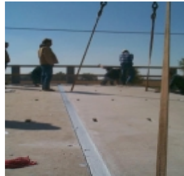
(b) Panels lowered into place
