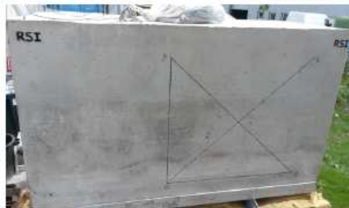
Figure 4. Cracking index measurements in the DEF mock-up
