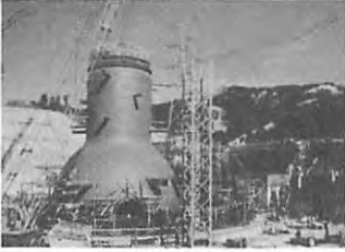
Fig 5.14 Drywell (JAPCO-1 TSURUGA)
