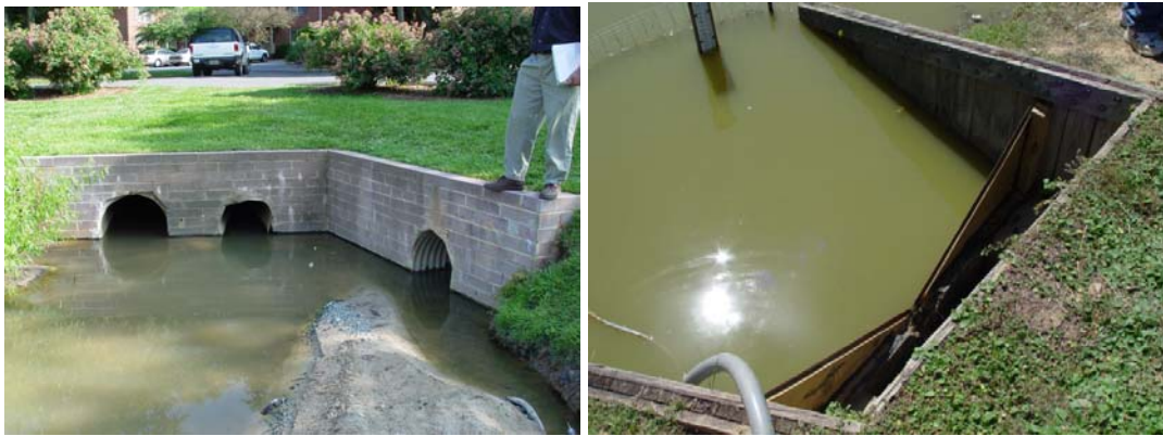
Figure 4.a and 4.b Locations of Inlet and Outlet Sample Collection
